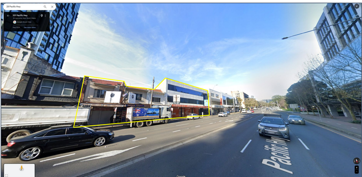
Figure 2.4 – Streetview image of the Pacific Hwy site frontage, looking west (Source: Google Maps)
